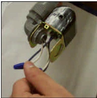
Straightening the wires
